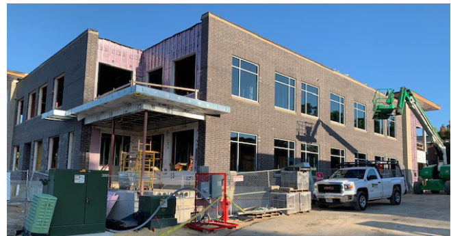
Construction of "Logic" by Stone House Development Inc.
