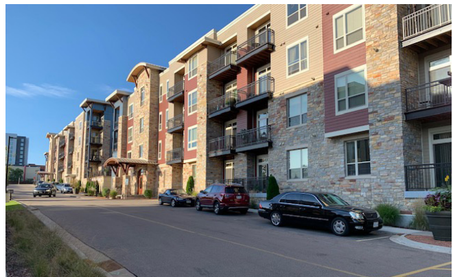
Completed Phase 2 of the Lodge at Walnut Grove.
